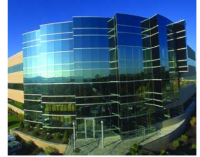
Graciano Brick Division's first job was the construction of the Graciano's new headquarters near Pittsburgh.
