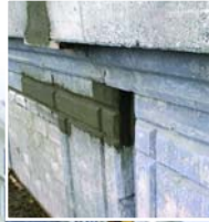
Shotcrete repair in progress.
