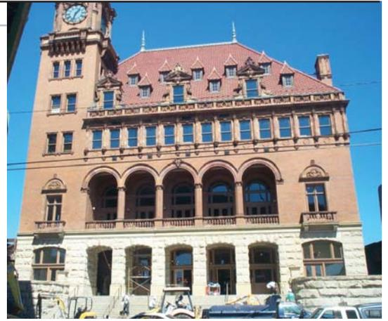
deteriorated significantly over time. Graciano launched a search among its stone suppliers and located stone that matched the original material in both color and texture at Waller Brothers Stone Company. Approximately 140 sections of stone were cut and tooled with grooves to match the architectural detail of the building.
